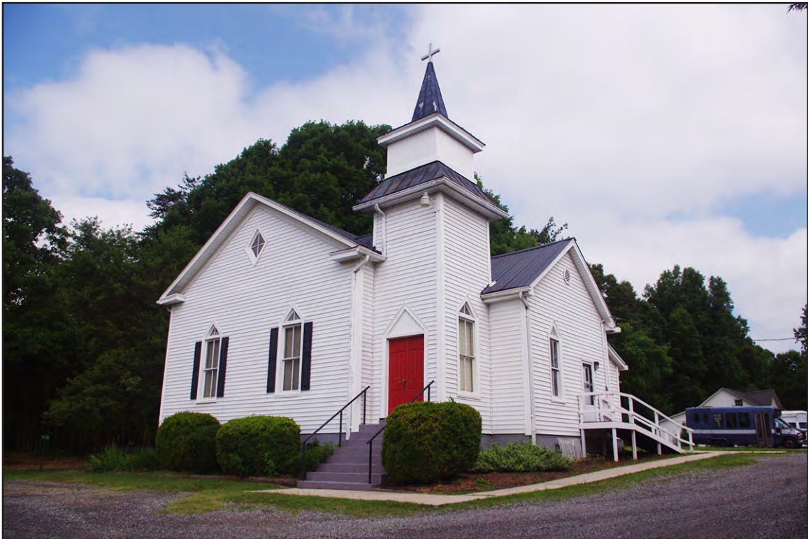
PLATE 29: Former Stoneville Methodist Church (RK1304), South and East elevations, Rockingham County, North Carolina
