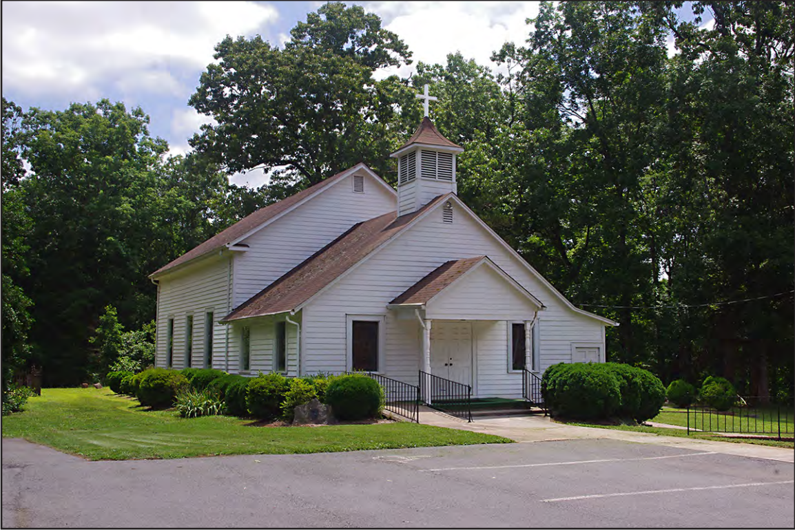
PLATE 34: Speedwell Presbyterian Church (RK0991), West and North Elevations, Rockingham County, North Carolina
