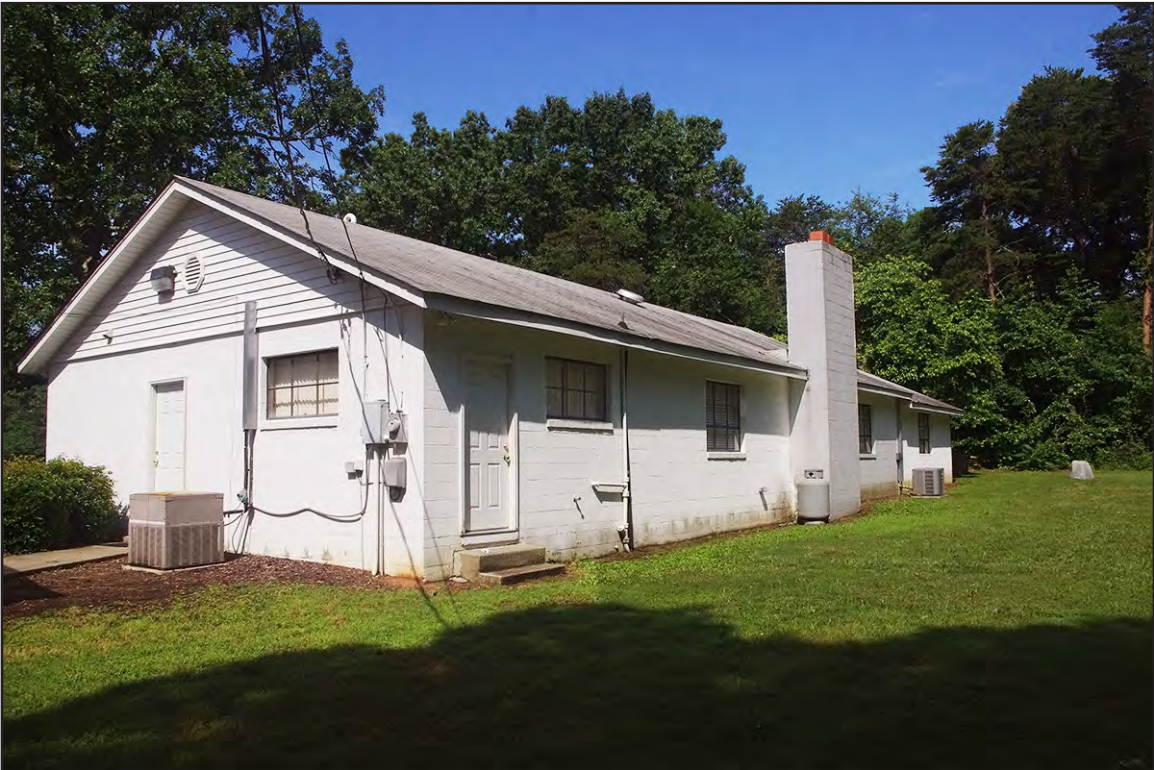
PLATE 16: East and North Elevations of Fellowship Hall, Mizpah United Methodist Church (RK1452), Rockingham County, North Carolina
