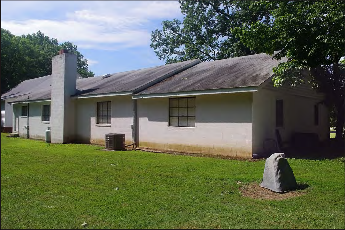
PLATE 15: Oblique View of North Elevation of Fellowship Hall, Mizpah United Methodist Church (RK1452), Rockingham County, North Carolina
