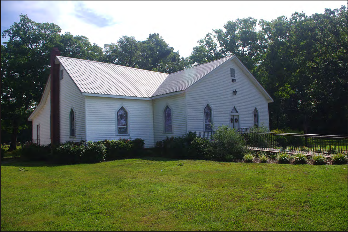
PLATE 3: South and West Elevations, Mizpah United Methodist Church (RK1452), Rockingham County, North Carolina
