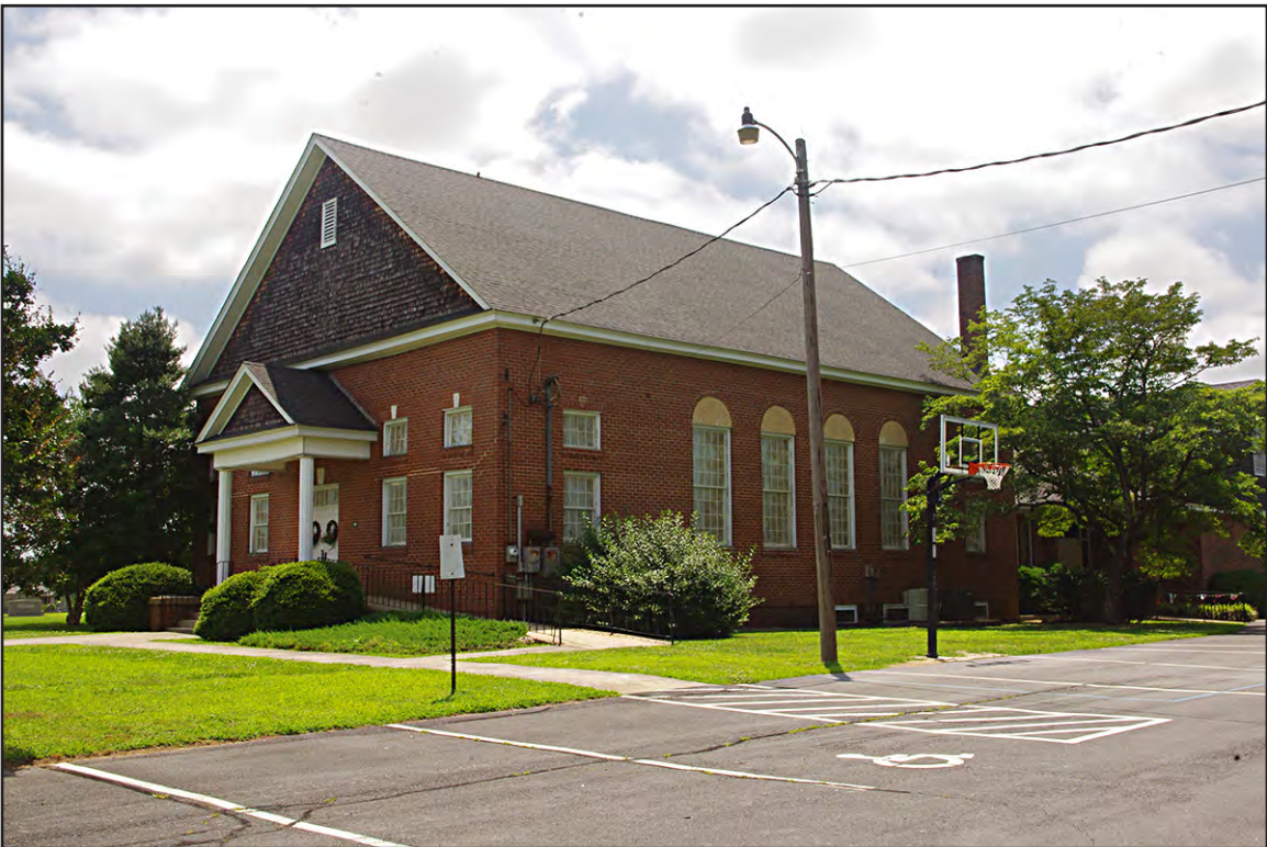
PLATE 31: Midway United Methodist Church (RK1346), North and West Elevations, Rockingham County, North Carolina
