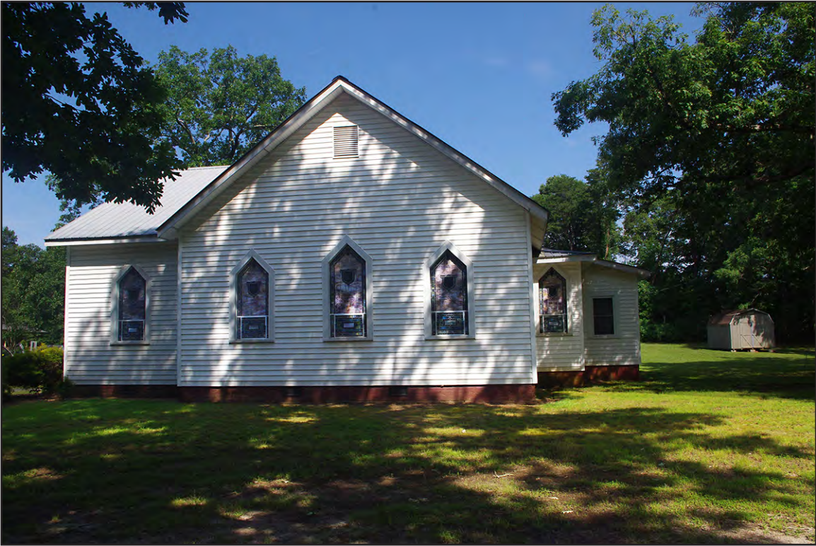
PLATE 5: East Elevation, Mizpah United Methodist Church (RK1452), Rockingham County, North Carolina
