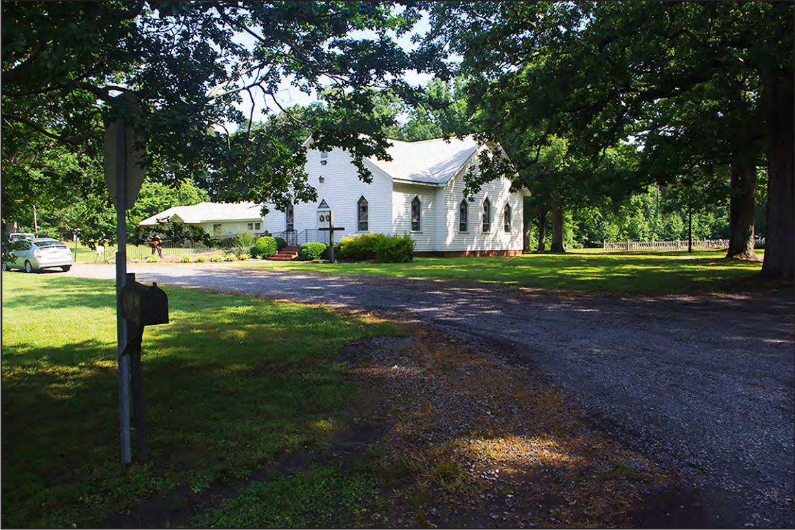
PLATE 1: Mizpah United Methodist Church (RK1452), Facing Northwest from East Side of Gravel Drive, Rockingham County, North Carolina
