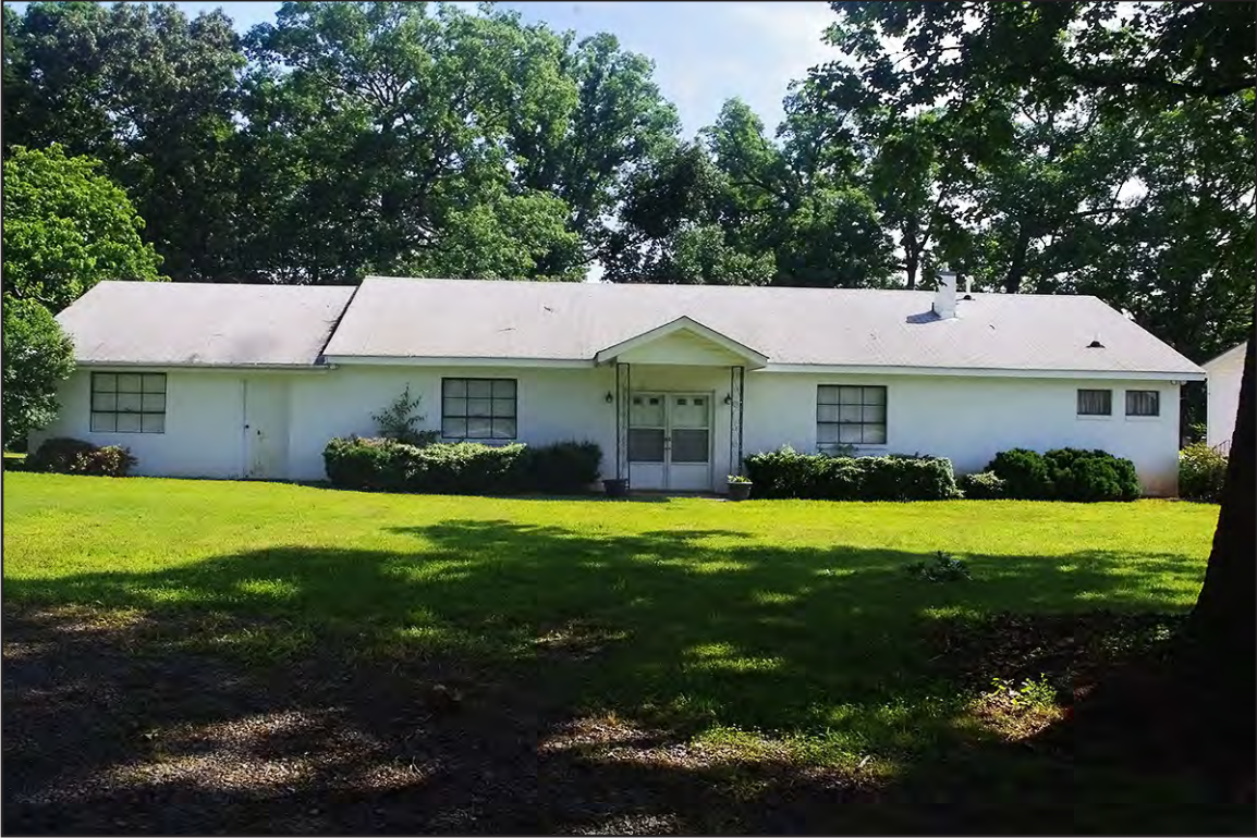
PLATE 13: South Elevation of Fellowship Hall, Mizpah United Methodist Church (RK1452), Rockingham County, North Carolina
